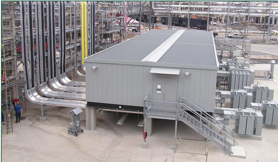
Power Control Room
