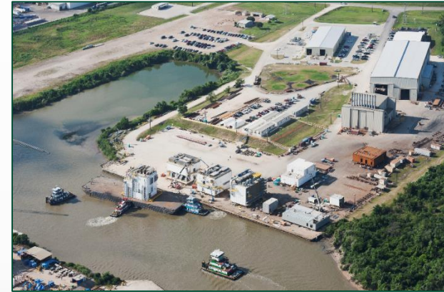
Jacintoport Blvd. Houston, Texas Office Fabrication Yard / 62 Acres 82,320 Square Feet Galveston Bay Access
