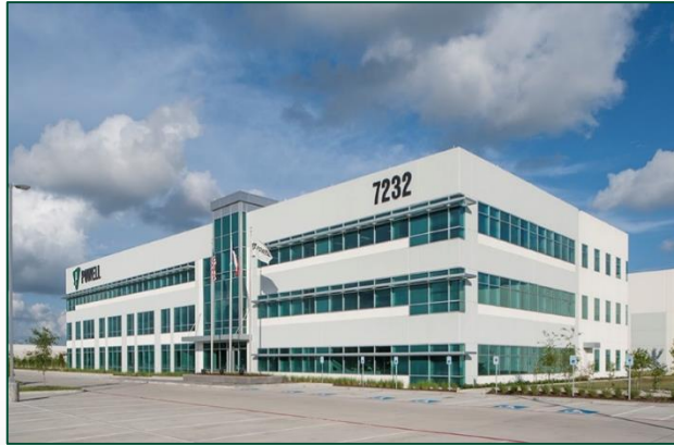
Airport Blvd. Houston, Texas Office Manufacturing Facility 290,554 Square Feet
